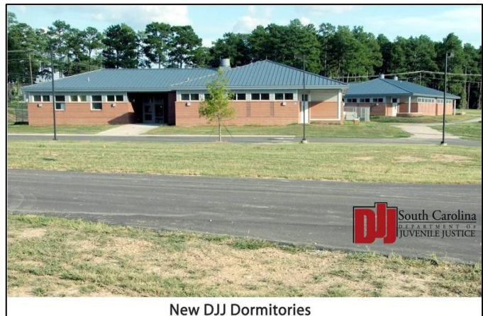
New DJJ Dormitories
